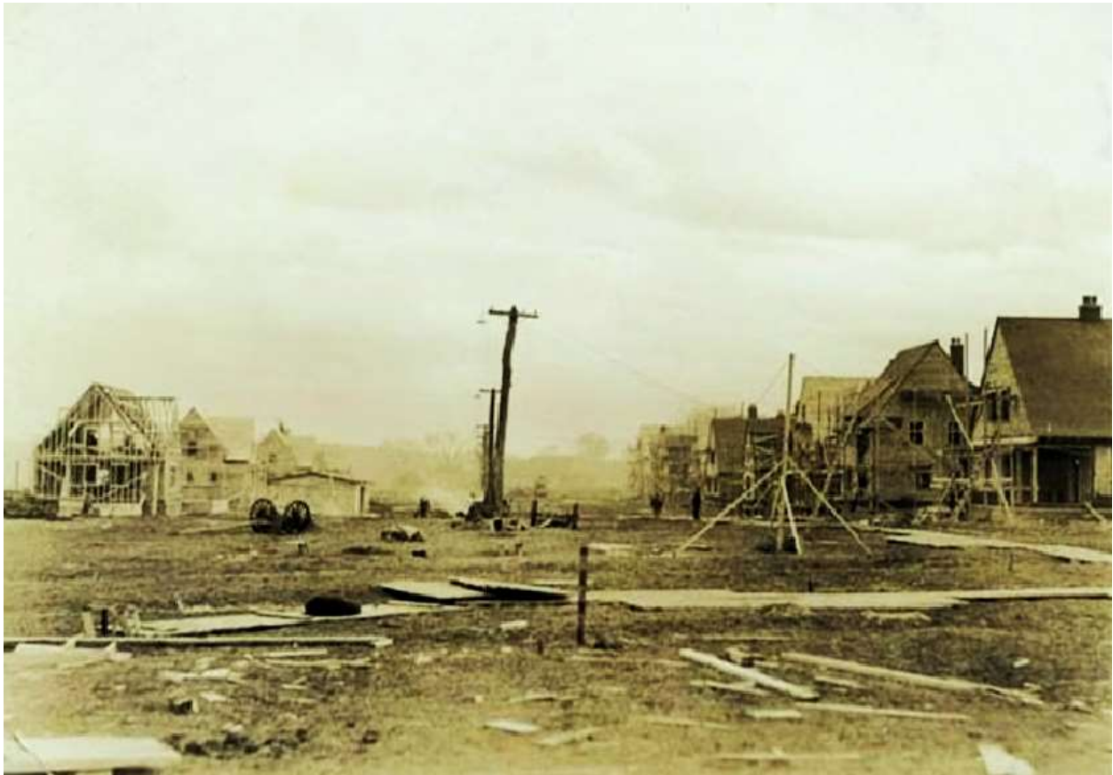
Figure 51 Gatineau Mills, Quebec, under construction, 26 October 1926.
