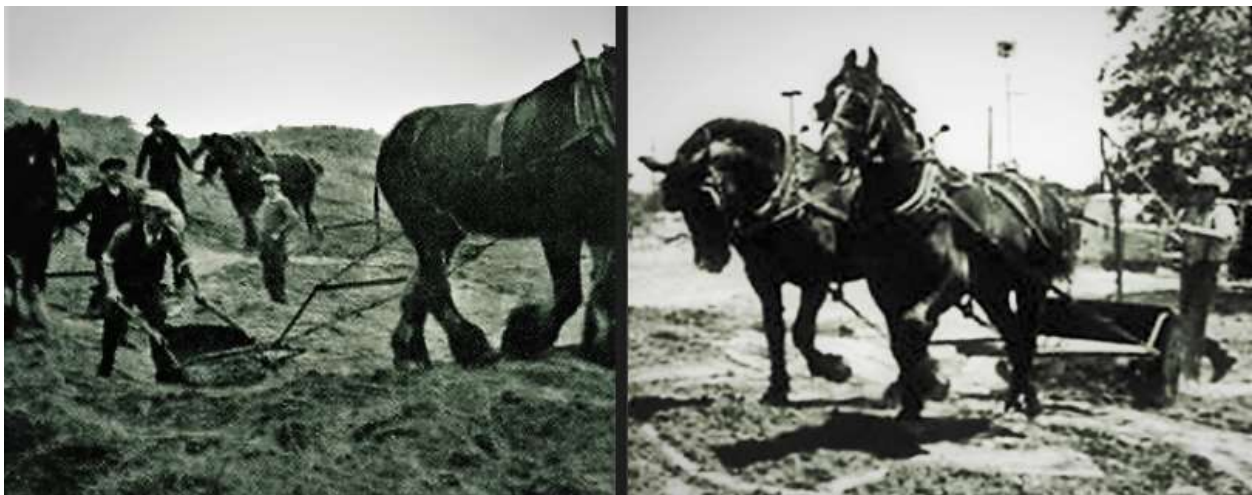
Figure 92 Left: teams with Fresno Scrapers circle around a green complex, scooping out soil from future bunkers and depositing the rough soil on the green site. Harry S. Colt and C.H. Alison, Some Essays on Golf Course Architecture (London: Country Life, 1920). Right: The operator of a Fresno Scraper lifts the handle upright to deposit its load on the green site, ready to pull the handle down again with a rope attached to it.
