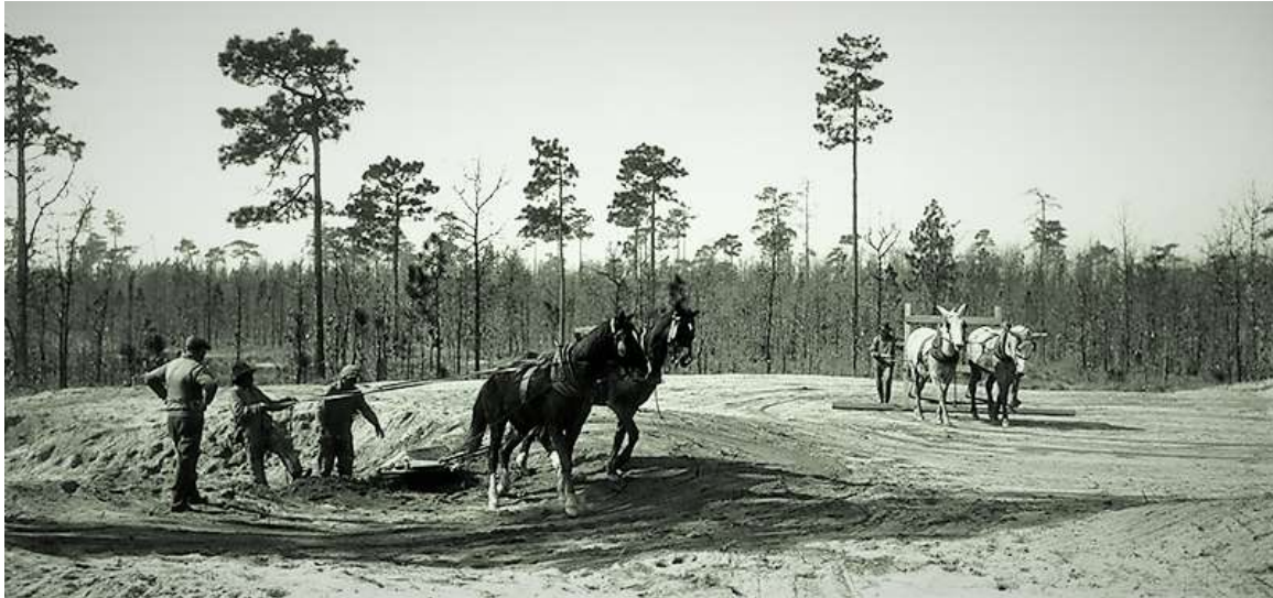
Figure 93 Fresno Scraper and Railway Plow operating in concert during green construction.
