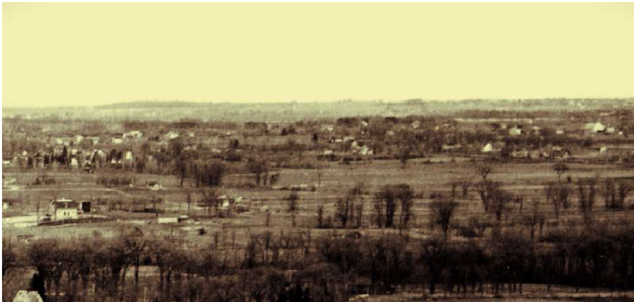
Figure 44 View of the McKellar Golf Club property circa April 1928. The clubhouse, under construction, can be seen on the left side of the photograph. The golf course land stretches to the right of the clubhouse.
