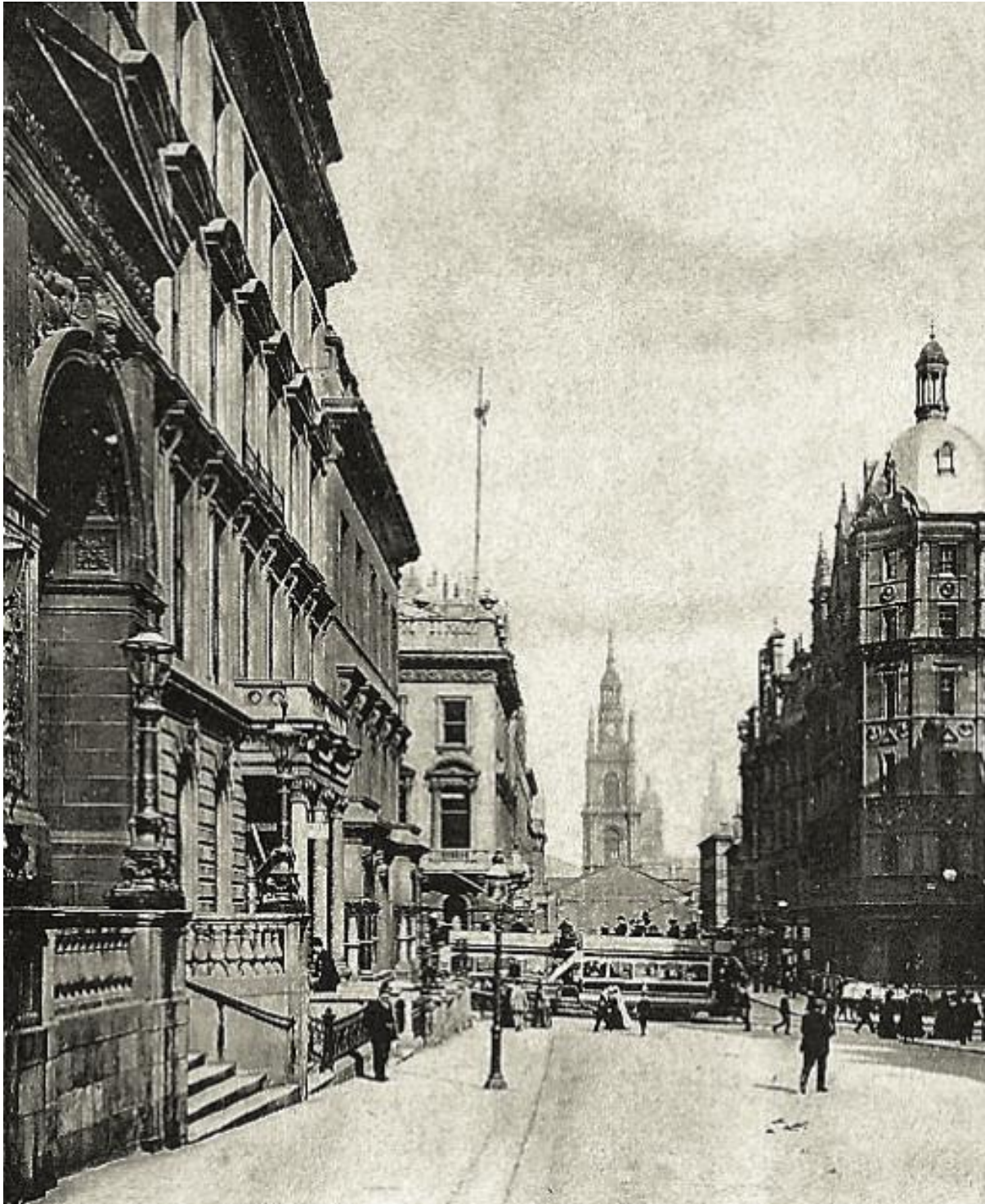
Figure 15 Glasgow's West George Street in the late nineteenth century. The photographer stands near Smith's apartment building at 145 West George Street.
