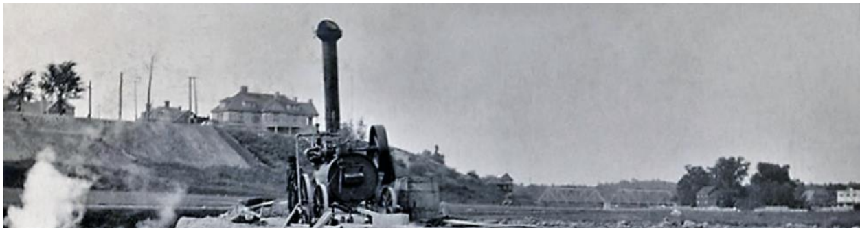
Figure 52 Cumming's Bridge and the home of Andrew W. Fleck at 500 Wilbrod Avenue are visible in the background of this 1904 photograph of construction work on Strathcona Park. The land is hardly above the level of the river. Henry Newell Bate funded this work to drain the swampy land of the Rifle Range to enable the building of Strathcona Park. Also visible in the photograph is the steep part of the Rideau bluff at the eastern end of the elevated ground on Sandy Hill.
