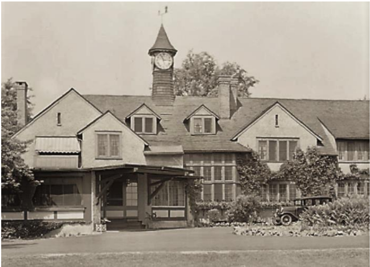
Figure 75 Country Club of Rochester shortly after its completion in 1903. It lasted until 1970.
