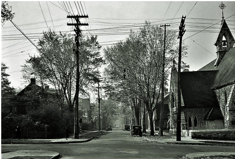
Figure 62 College Avenue at Laurier Avenue East (formerly Theodore), early twentieth century.
