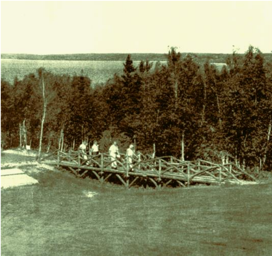
Figure 15 The "rustic bridge, built from natural twisted limbs of poplar and willow." Waskesiu Golf Course website photograph, 2023.
