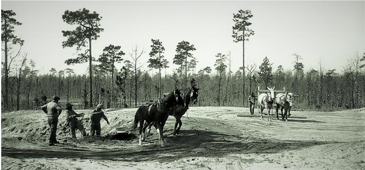
Figure 99 Teams scooping rough soil out of a bunker site with a Fresno scraper and smoothing the green surface with a Railway Plow.
